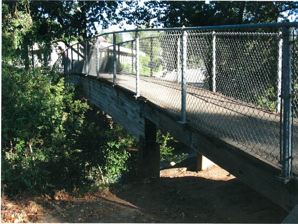
Figure 5. Existing Library Bridge, From Left Bank
