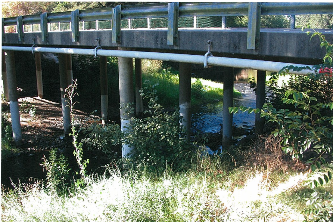
Figure 2. Folsom Road Bridge, Looking Upstream from the Left Bank
