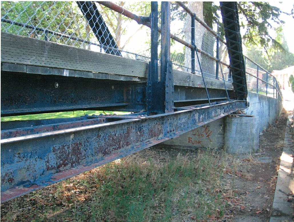
Figure 4. Ice House Bridge, Abutment on Left Bank
