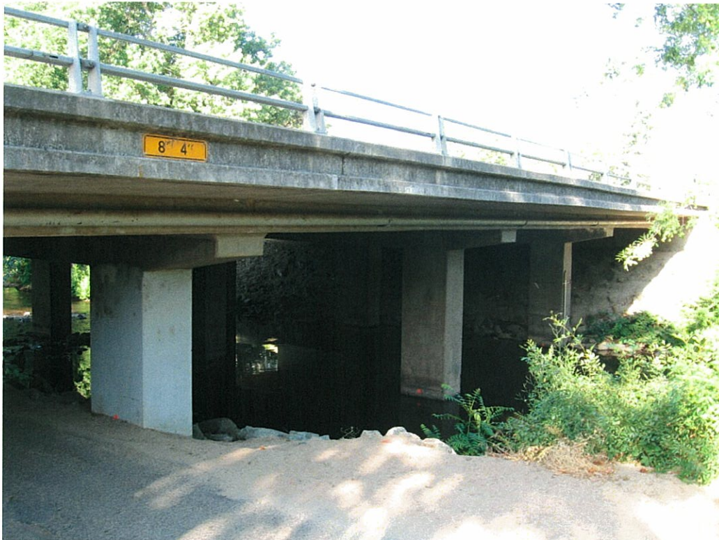
Figure 6. Douglas Boulevard Bridge, Looking Downstream from the Left Bank
