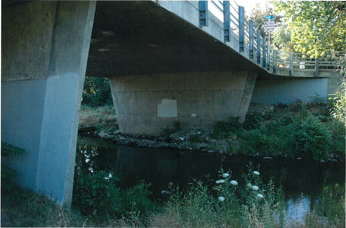
Figure 3. Lincoln Street Bridge, Downstream to the Left
